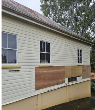
St Matthew's Hall renovations and new chairs
